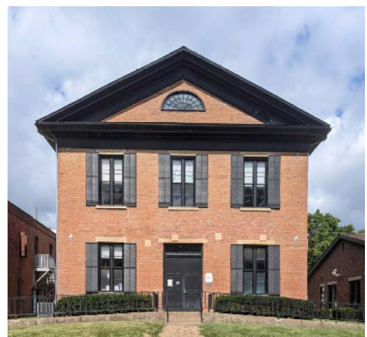
Van Buren County's Greek Revival style courthouse is Iowa's oldest courthouse in continuous use. The Great Places committee has identified the restoration of this building as a priority project. (courtesy of Paul Larson, Van Buren County Historic Preservation Commission)
